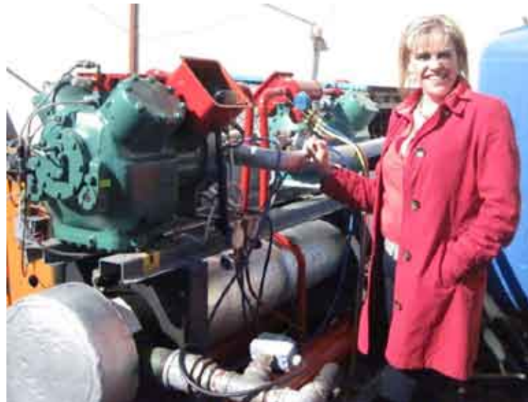
Carrier Water Cooled Chiller 110kw
